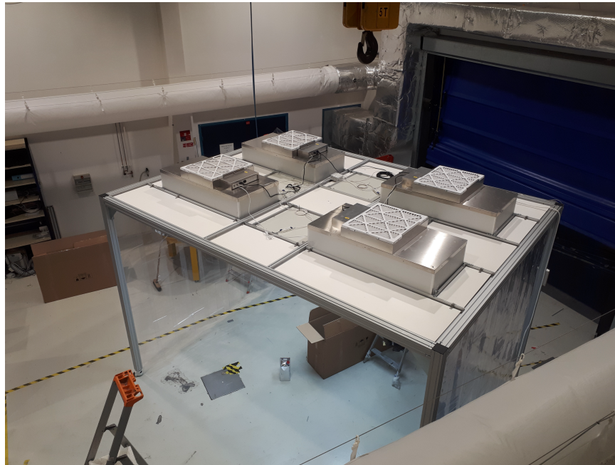
Figure 12: cleanroom is building inside the integration hall at IPAG. (2021 January)
